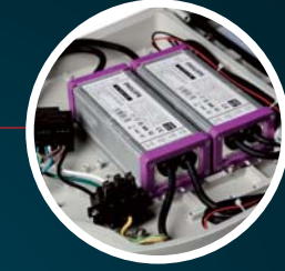
LED driver with a wide range of control and driver current options
